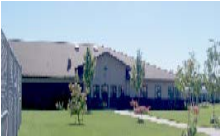
Clark County Work Release
