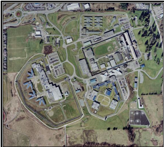
MCC Aerial View
