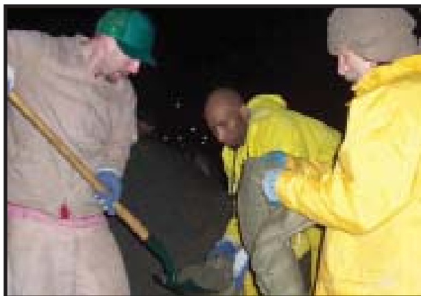
Sandbagging in Snohomish: Offender work crews from Monroe Correctional Complex filled sandbags and helped prevent flooding in Snohomish County.
