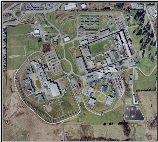
MCC Aerial View
