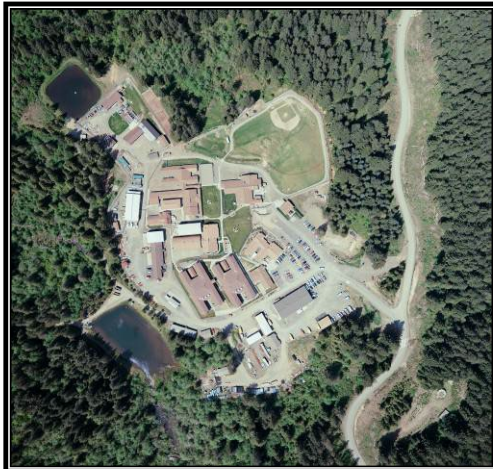
LCC Aerial View
