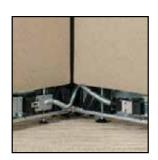
Panel electric conversion jumpers convert the old electrical 8-wire system to the new Universal electrical system.
