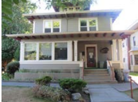
Rap House / Lincoln Park Work Release
