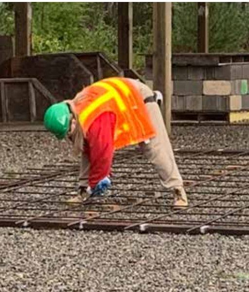
AMBER FISHER PREPARING REBAR
